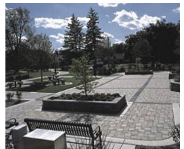
Pavers with concrete bands
