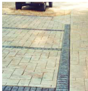
Concrete scored in a pavement pattern
