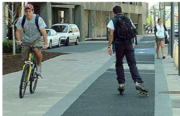
Bituminous and paver multi-use path
