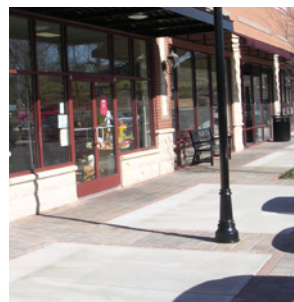
Concrete and paver sidewalk
