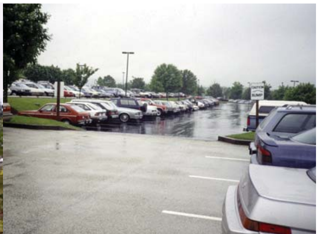
Example of a commercial parking lot utilizing porous pavement.
