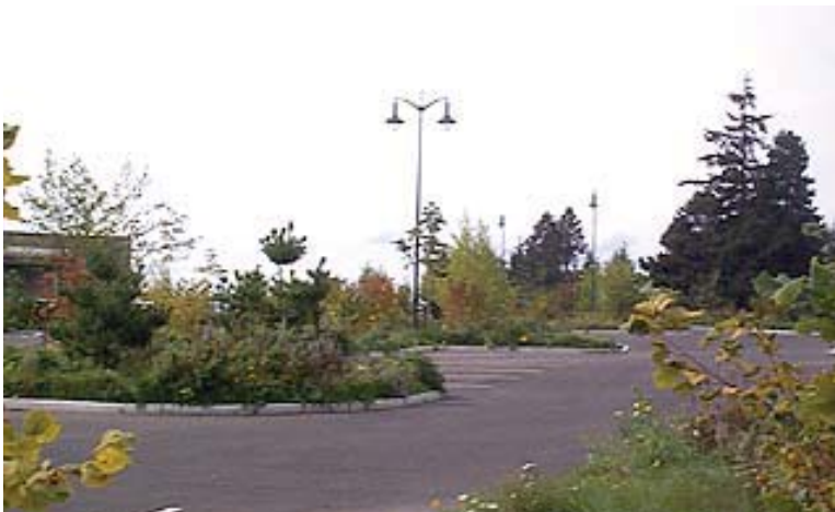
Example of bioretention basins/rain gardens within a commercial parking lot.
