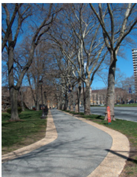
Bituminous path with exposed aggregate concrete edge
