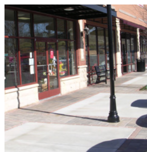
Concrete and paver sidewalk
