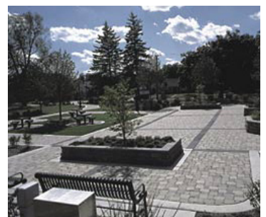
Pavers with concrete bands
