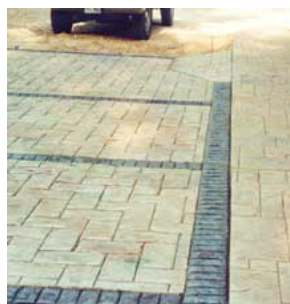
Concrete scored in a pavement pattern
